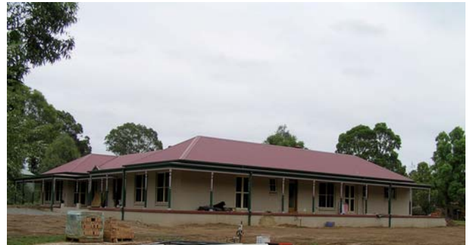
Above: view of the residence, during the final stages of construction
